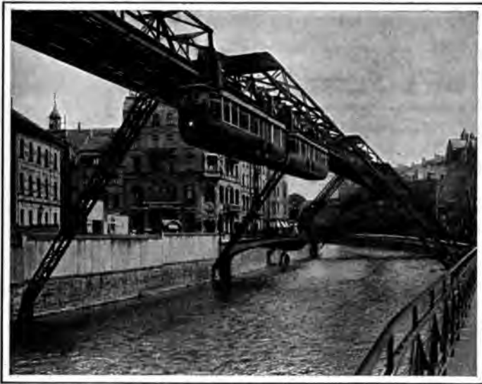
55. THE SUSPENDED TRAMWAY AT BARMEN-ELBERFELD. — One of Germany's engineering triumphs.
